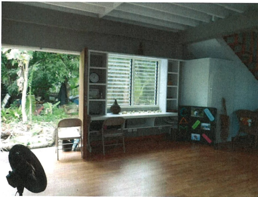
Inside view of the first floor of the Training Center
