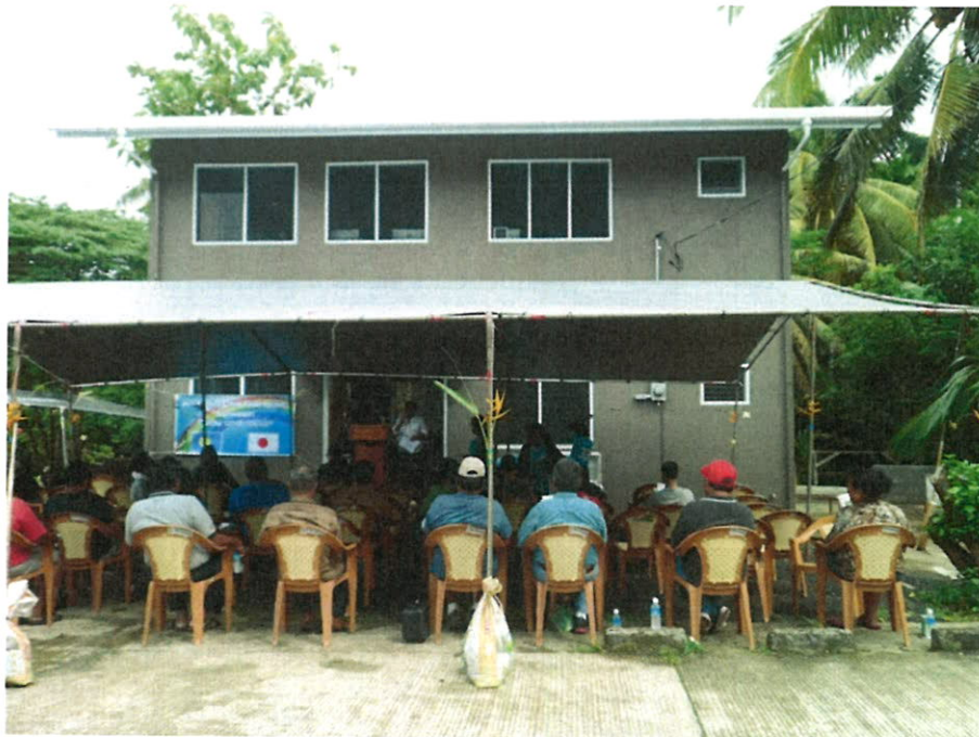
View of the front of the Training Center
